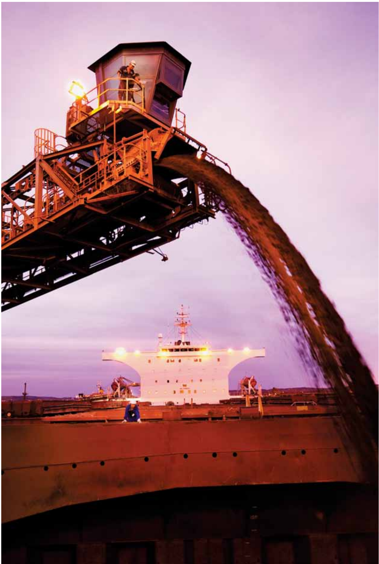
Loading a ship at Parker Point iron ore terminal.
