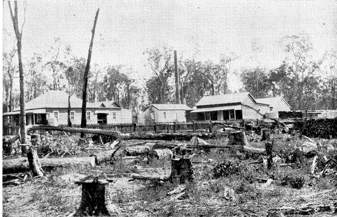
GENERAL VIEW, GREENBUSHES TIN SMELTING WORKS.
