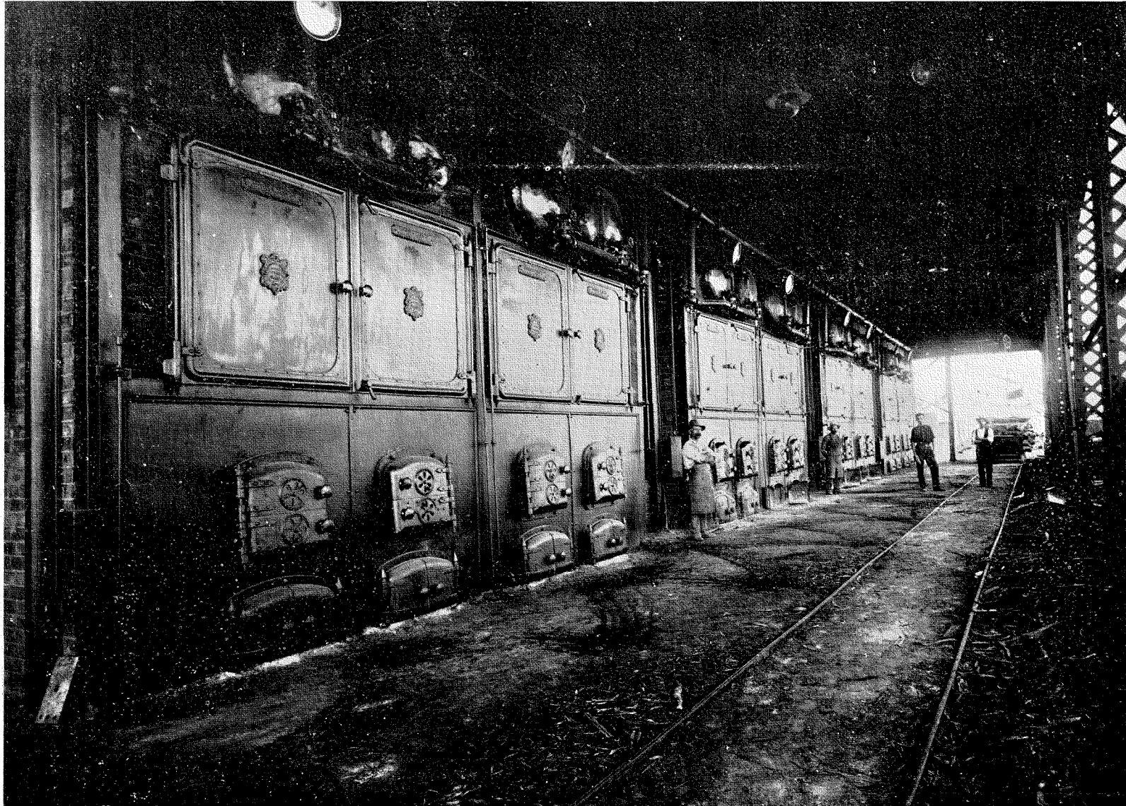
KALGOORLIE ELECTRIC LIGHT AND POWER CO.'S STATION, KALGOORLIE. (East Coolgardie Goldfield.)
