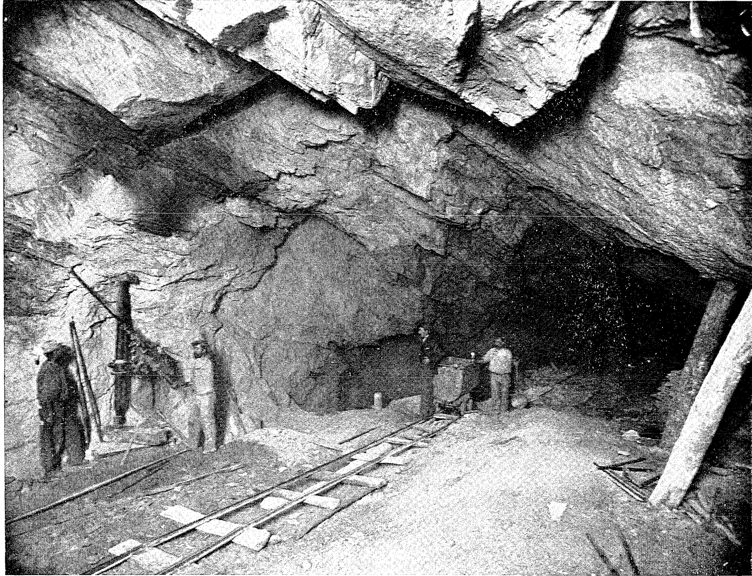
UPPER STOPES BETWEEN NO. 4 LEVEL AND NO. 5 LEVEL, BROWN HILL G.M., KALGOORLIE. ( East Coolgardie G.F. )
