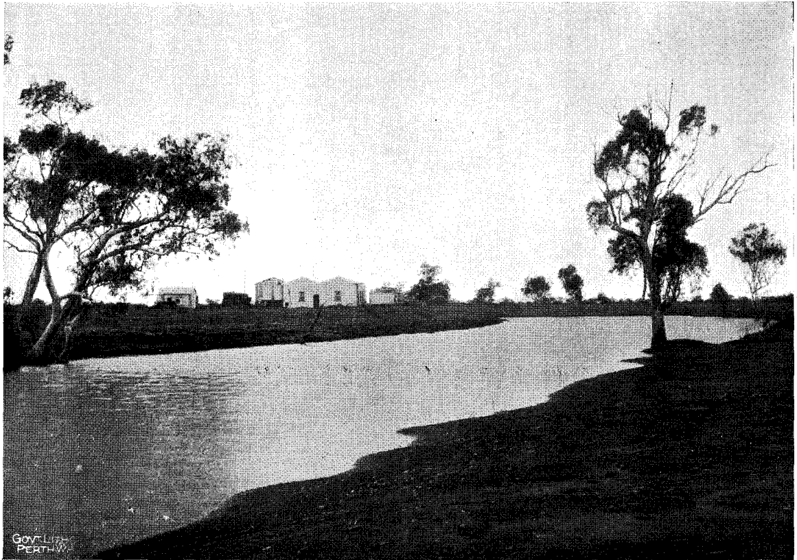
LEONORA WATER SUPPLY. Pump Station and Reservoir, 10 miles north of Leonora. Capacity, 14 million gallons (after rain).
