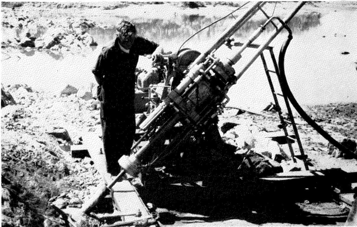
Petrol Rig Showing Anchor Bolts. Site D.D.H.3B.
