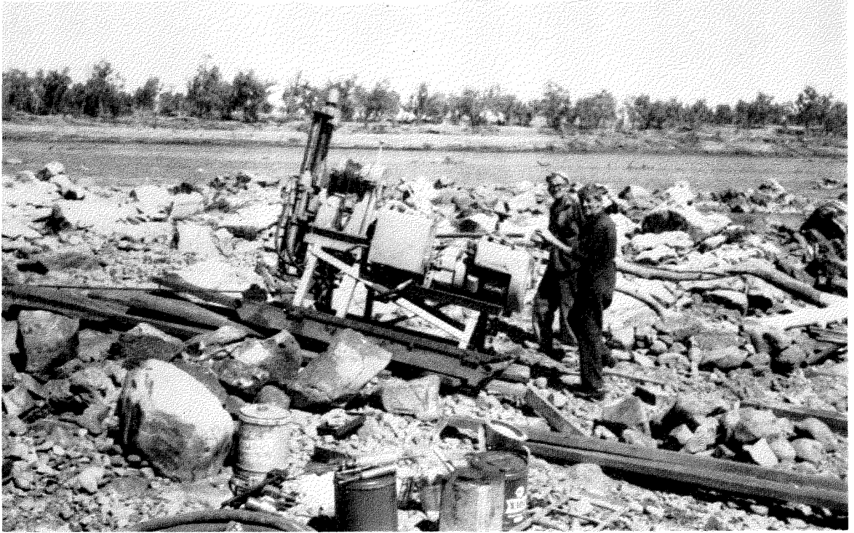
Shifting Petrol Rig Over Typically Rugged Surface of Bandicoot Bar.
