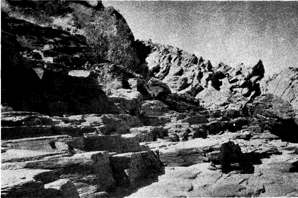
Fig. No. 4.—Northern Spillway looking East. Faulted contact between Quartzite Phyllite showing blocky characteristics of Phyllite.
