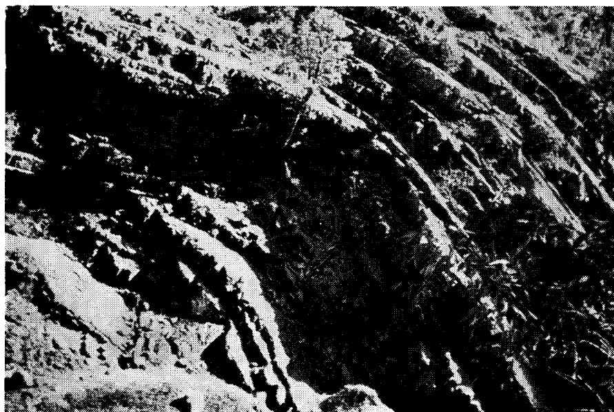
Fig. No. 12.—East Abutment looking North East showing quartzite steepening in dip.
