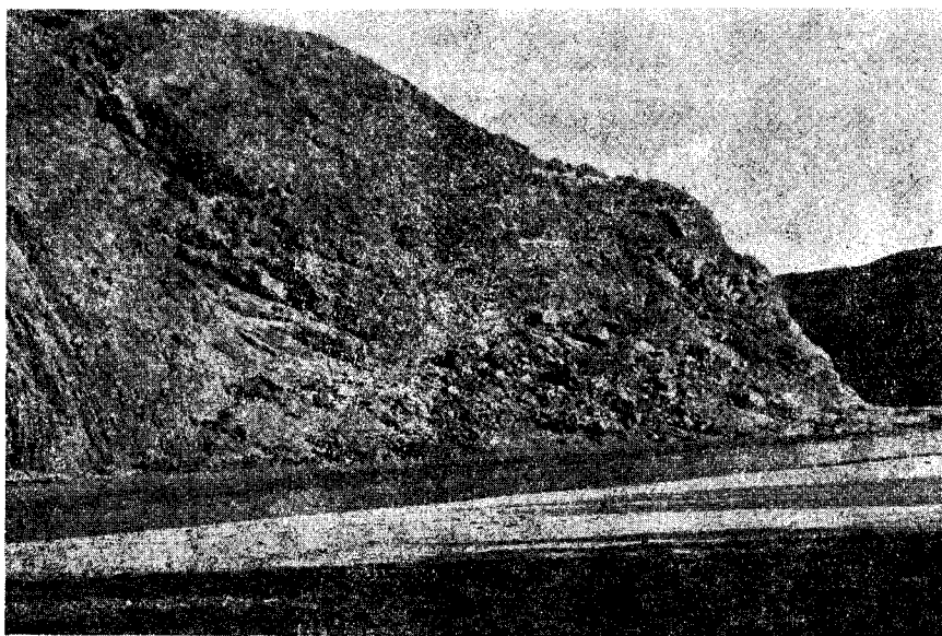
Fig. 5. West abutment showing "notch" area.
