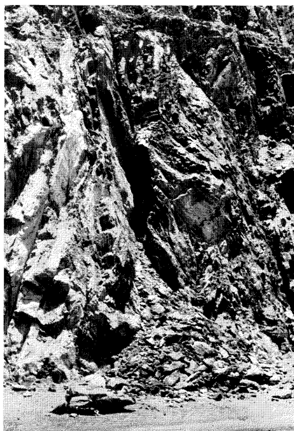
B—North wall between 22 miles 04 chains and 05 chains. Overshot toe has given an almost vertical face in folded, jointed and weathered amphibolite. Rock falls of minor size are to be expected with further weathering. Rafts of granite are notable. (F891)
