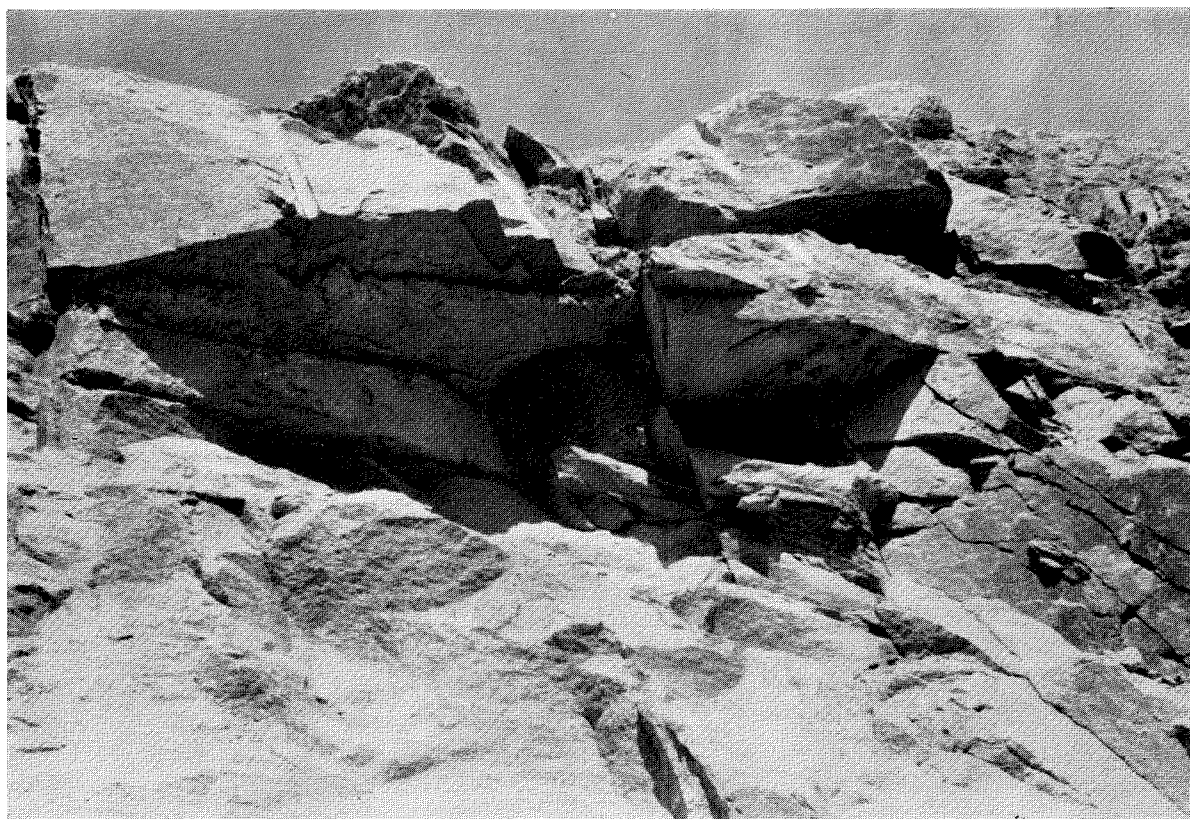
A—Overhangs caused by the presence of sheet joints channelling blasting. A weathered clay seam on a sheet joint 6 inches thick is seen immediately under the main overhang ; F 1155.
