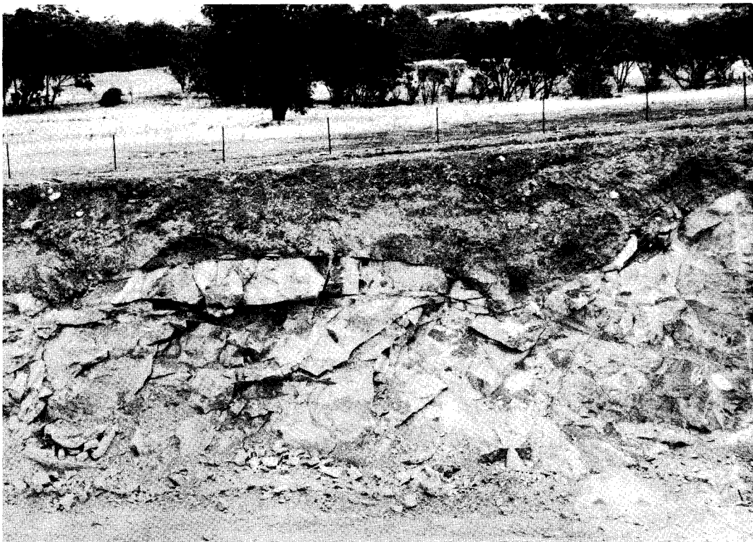
B. Prominent sheeting causing large overhangs after blasting. Abrupt transition from weathered to fresh rock because of control of water movement on the top sheet joint; FN 1240.
