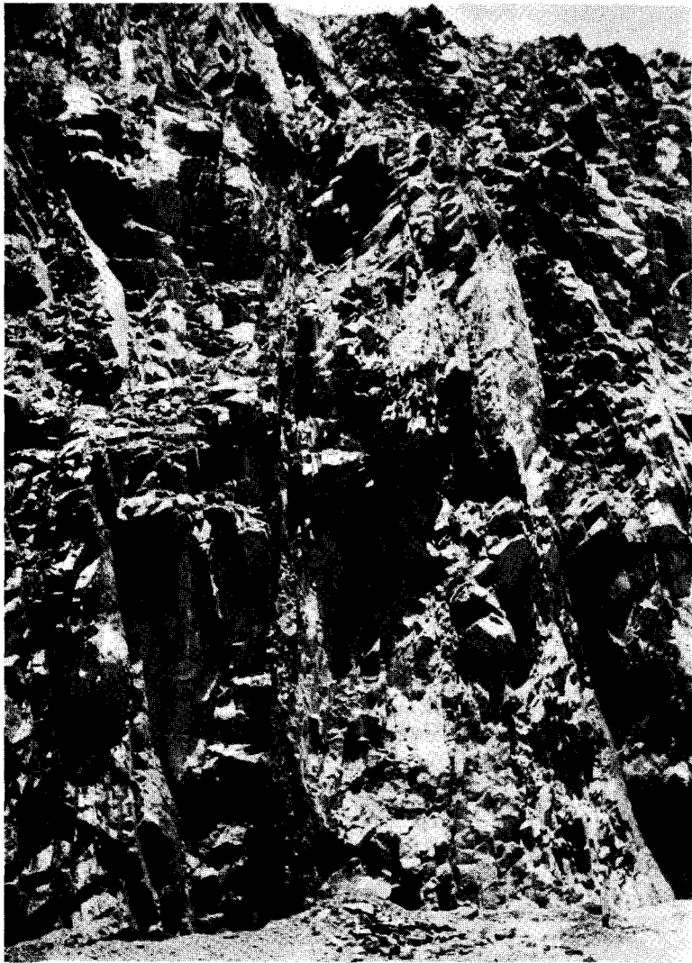
A. Overbreak caused by the channelling effect of open cross joints, in this case foliation joints; FN 1239.
