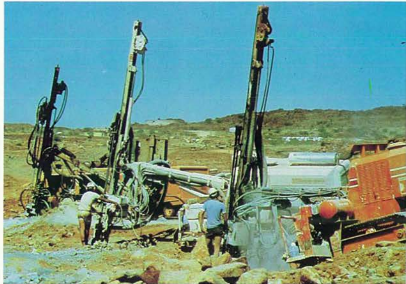
Drilling blast holes.
