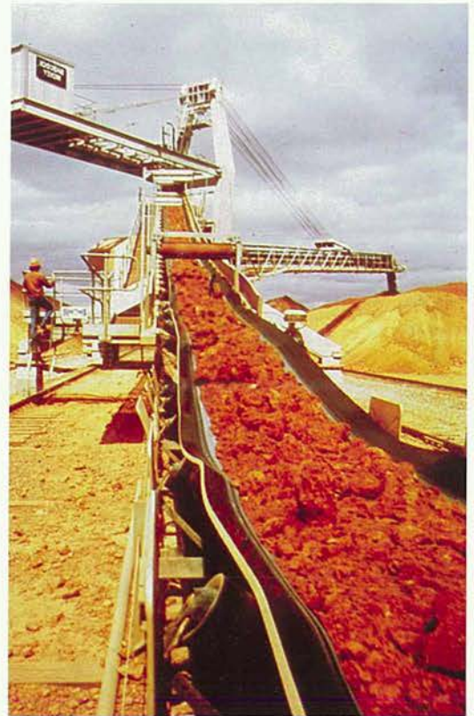
Belt conveyor shifting bauxite.
