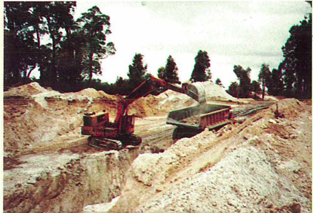
Typical mining operation in weathered pegmatite at Greenbushes (Greenbushes Tin N.L. photo).
