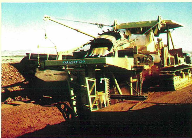
Digging the trench for the Dampier-Perth Gas Pipeline.
