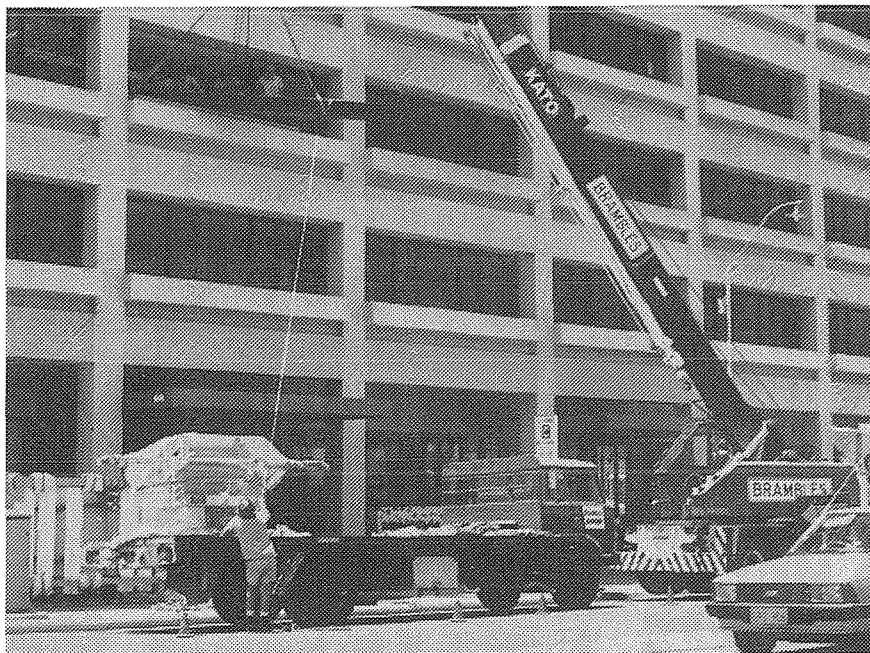
Installing the OPTI COPY process camera in the Surveys and Mapping Division photo-process laboratory, Mineral House.
