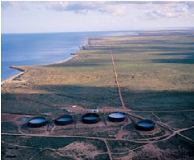
BARROW ISLAND, PROPOSED SITE FOR GORGON PROJECT GAS PROCESSING FACILITY (PICTURE COURTESY OF CHEVRON)
