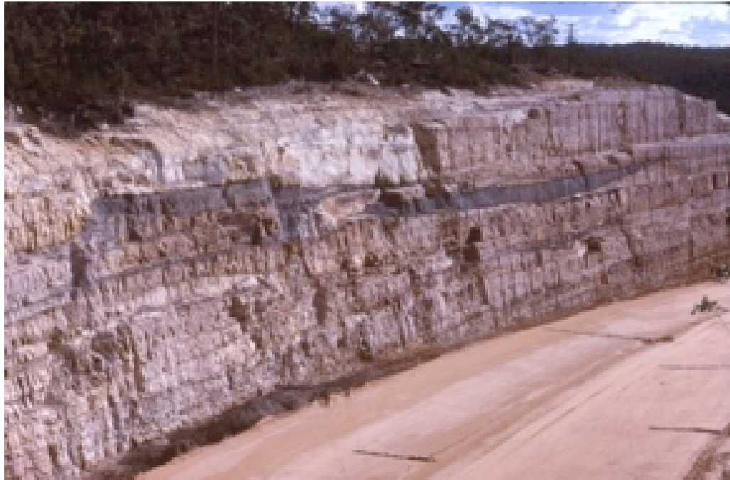
Figure 5.5: Pacific Hwy cutting near Gossford through Triassic Hawkesbury Sandstone. Photo courtesy of J Roestenburg (Roestenburg, 2016).
