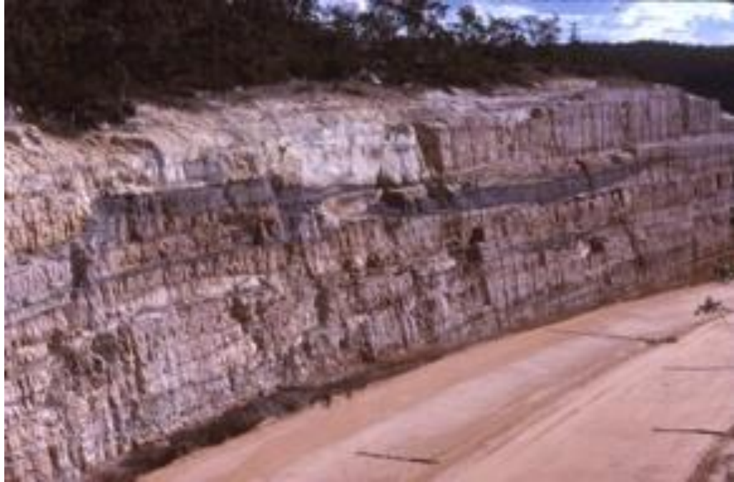
Figure 5.10: Pacific Hwy cutting near Gosford through Triassic Hawkesbury Sandstone. Photo courtesy of J Roestenburg.
