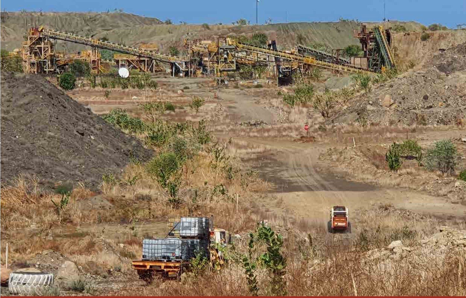
Image 4 – Removal of hydrocarbons and waste containers from the E9 area
