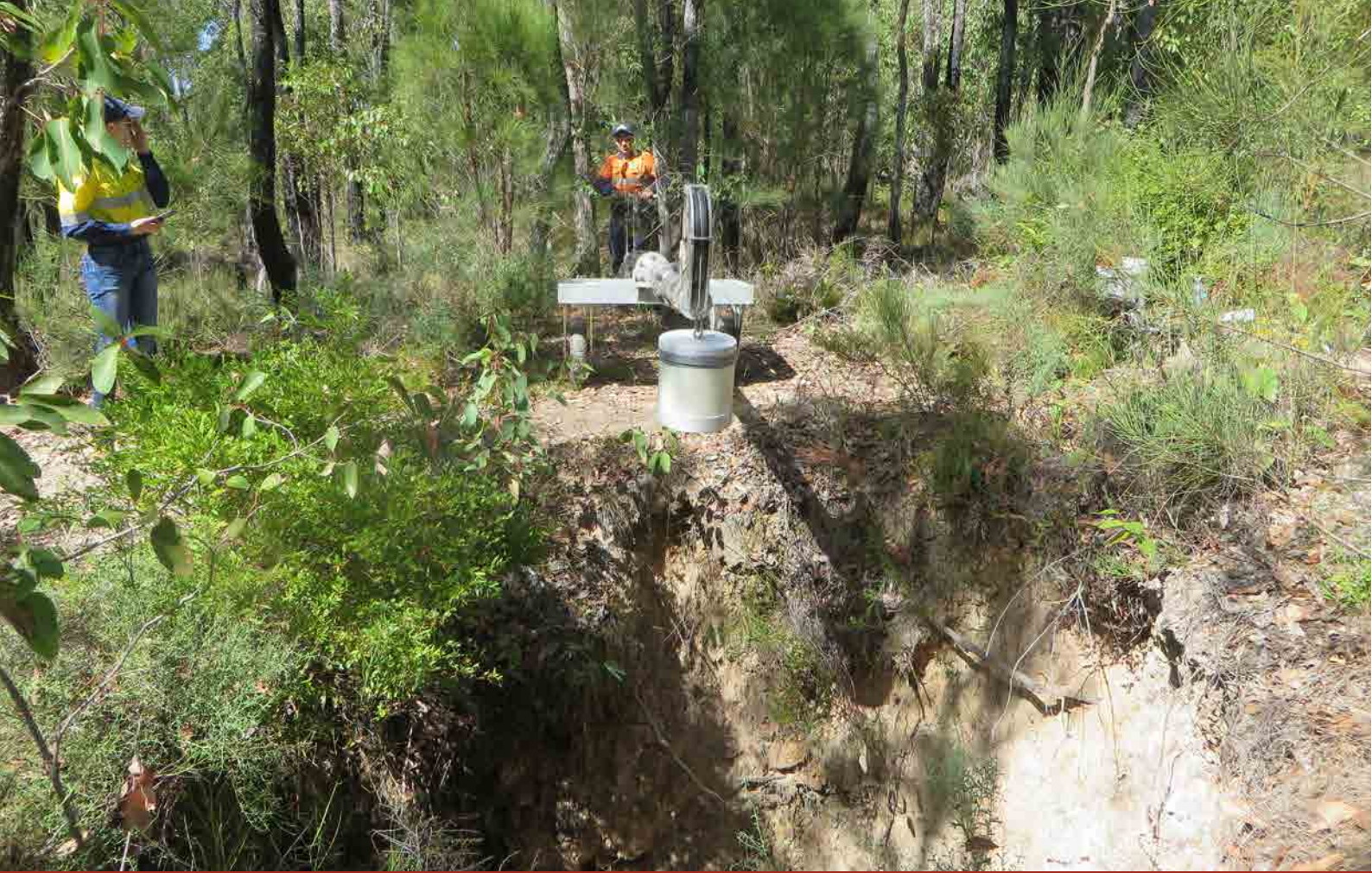
Image 3 – Geotechnical assessment down shaft camera and LiDAR survey
