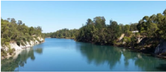
Figure 9: Steep unstable pit wall along southern side of Black Diamond pit lake.
