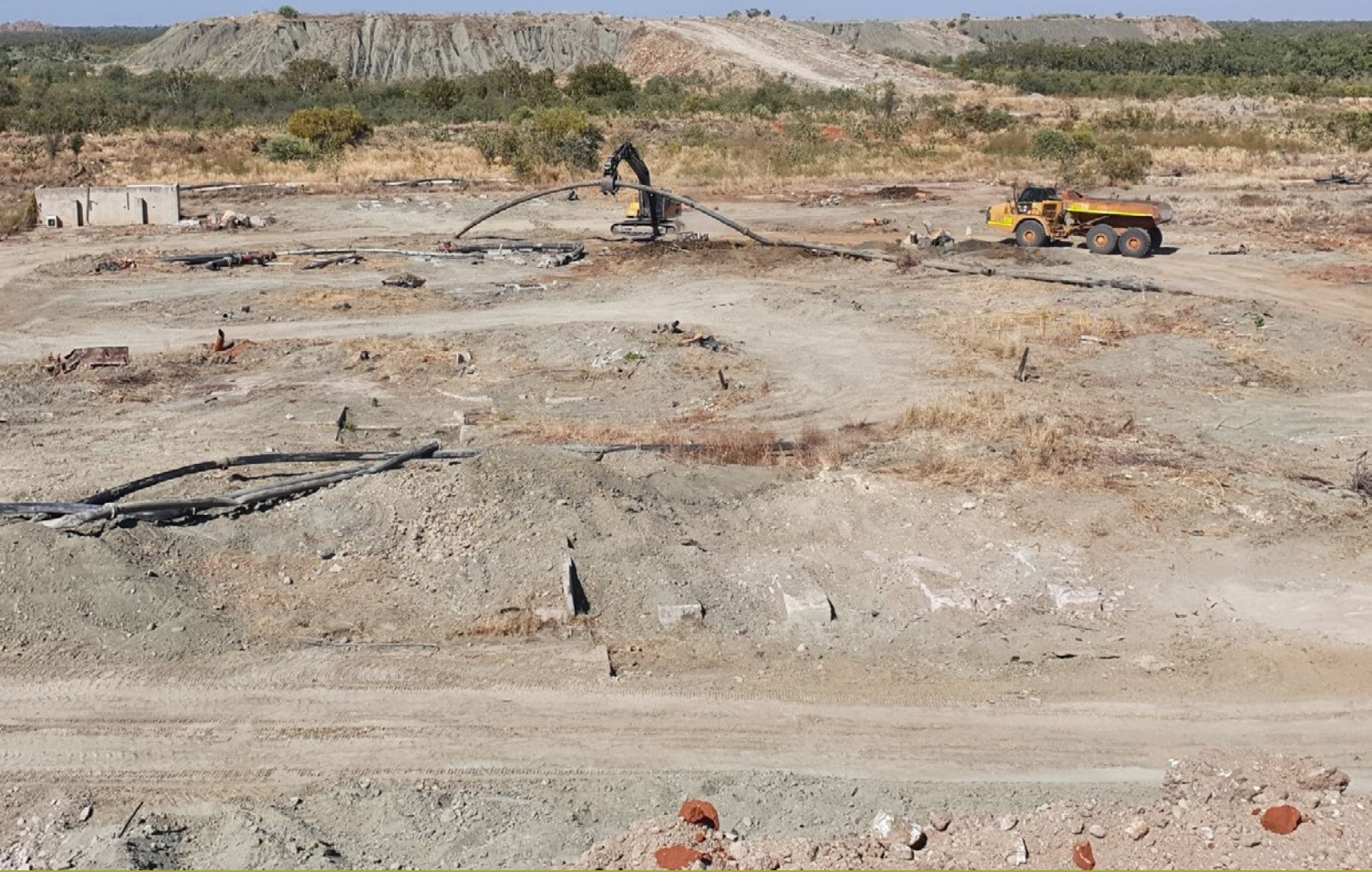
Image 3 – E9 plant area works continuing post removal of redundant infrastructure
