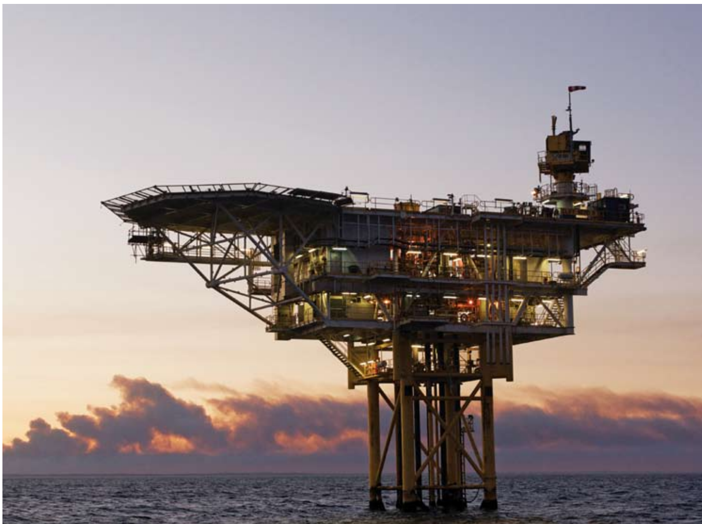
The Blacktip platform in WA-33-L (Photo courtesy of ENI)
