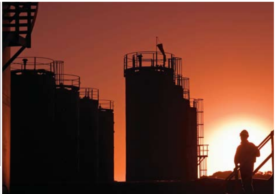
Hovea production facility (Photo courtesy of ARC Energy)
