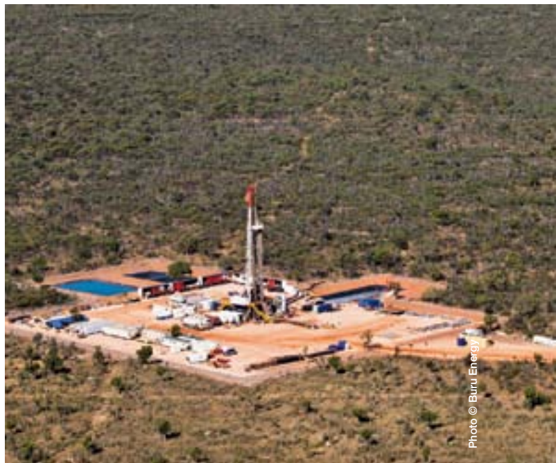
A Buru Energy gas site development
