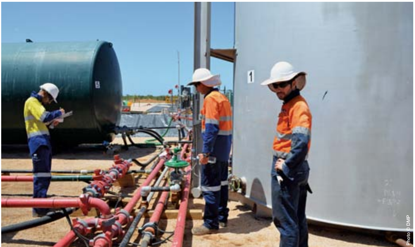
DMP inspector auditing the Ungani facility
