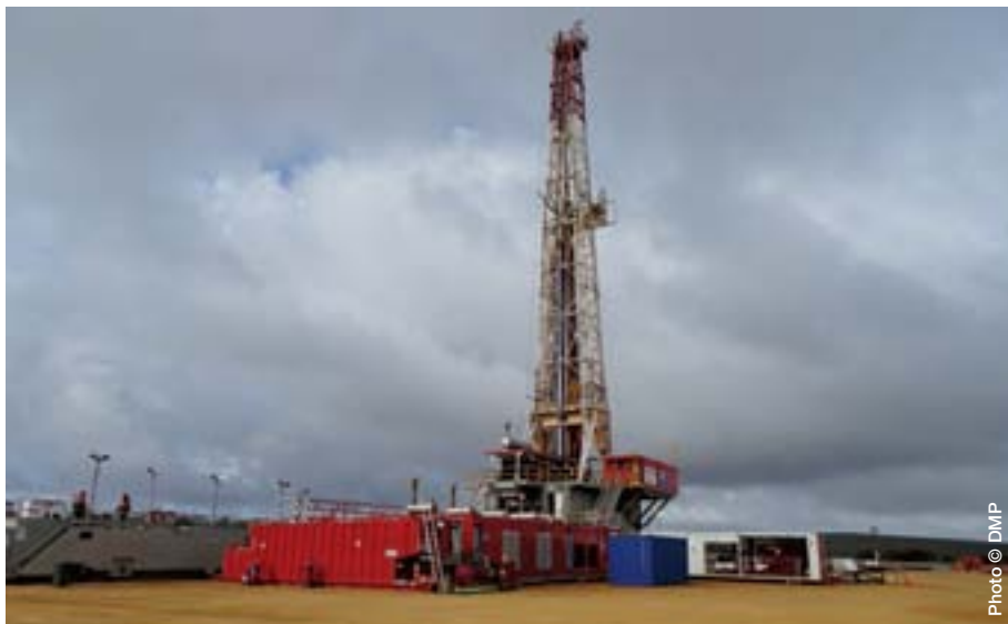
Energdrill rig 3 at Drover 1 in the northern Perth Basin
