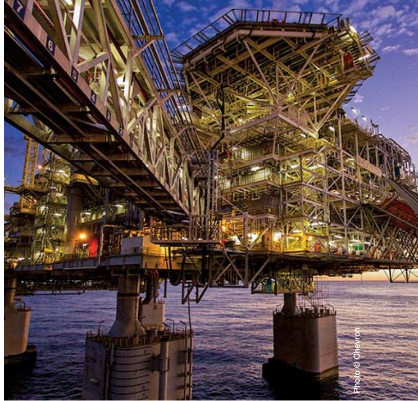
Hook up and commissioning underway at the Wheatstone Platform
