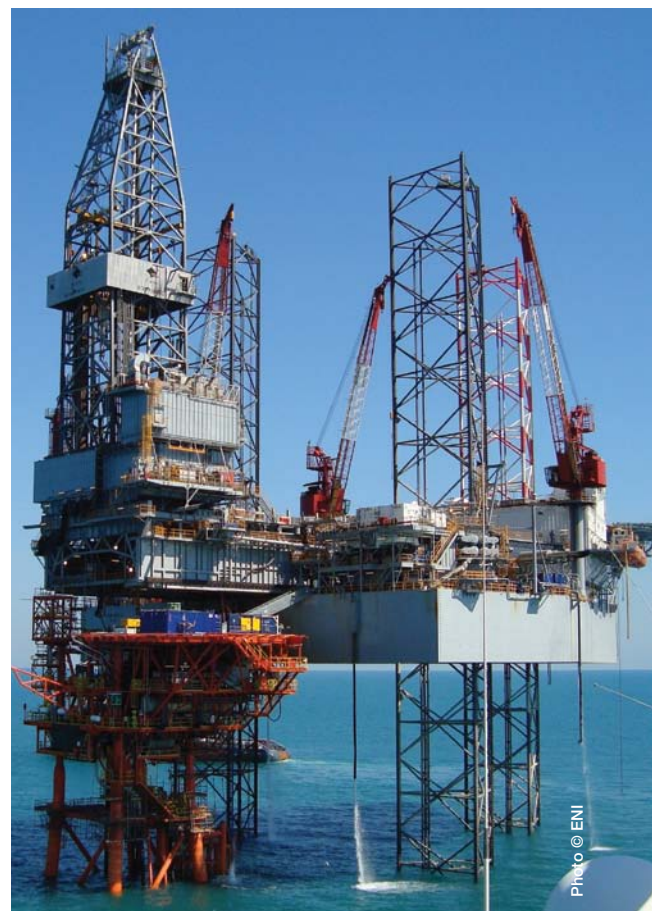
Jackup rig at the Blacktip platform
