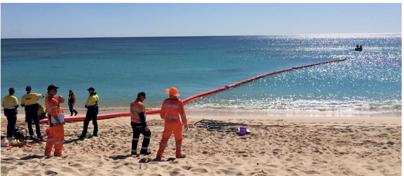
Deployment of shoreline protection boom
