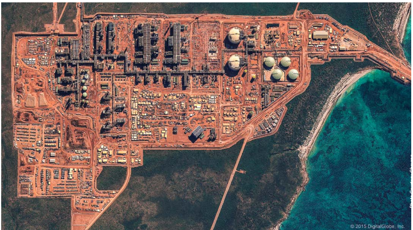
Aerial view of the Gorgon Project on Barrow Island
