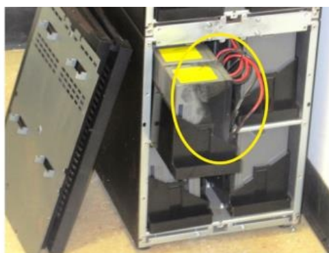
UPS battery cabinets. Left. Potential for inadvertent access as indicated by arrow. Right. Exposed live terminals (arc flash damage indicated by circle).
