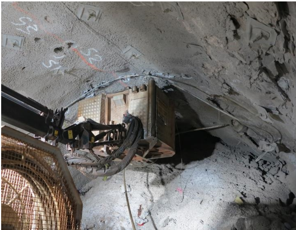
Charge-up basket near the roof of the cross-cut
