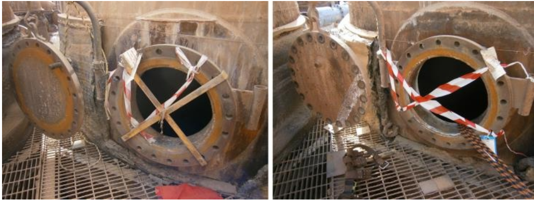
Left: Manway into a digester with mechanical guard fitted. Right: Manway entry for the digester without scaffolding (tape placed by emergency response team).
