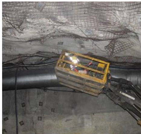
IT work basket in position beneath the backs
