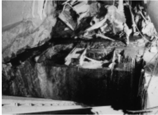
580m level Plat, looking down the shaft, at Peterson #2 sub-incline rock shaft
