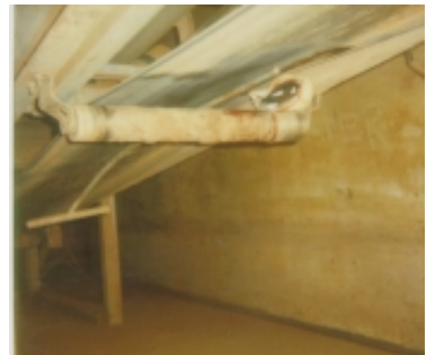
Accident scene showing entry point, scraper and helmet
