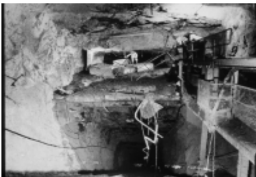
580m level Plat, looking down the shaft at Peterson #3 man/materials sub-incline shaft
