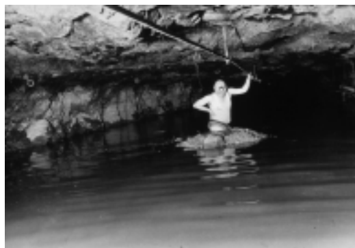
Typical main haulage (8m x 4.5m) after the mudrush
