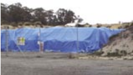
Ammonium nitrate storage
