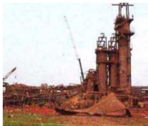
Gramercy Digestion plant - after explosion
