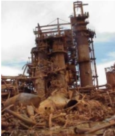
Total destruction of digestion plant area
