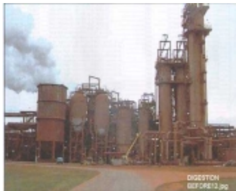
Gramercy Digestion plant - before explosion
