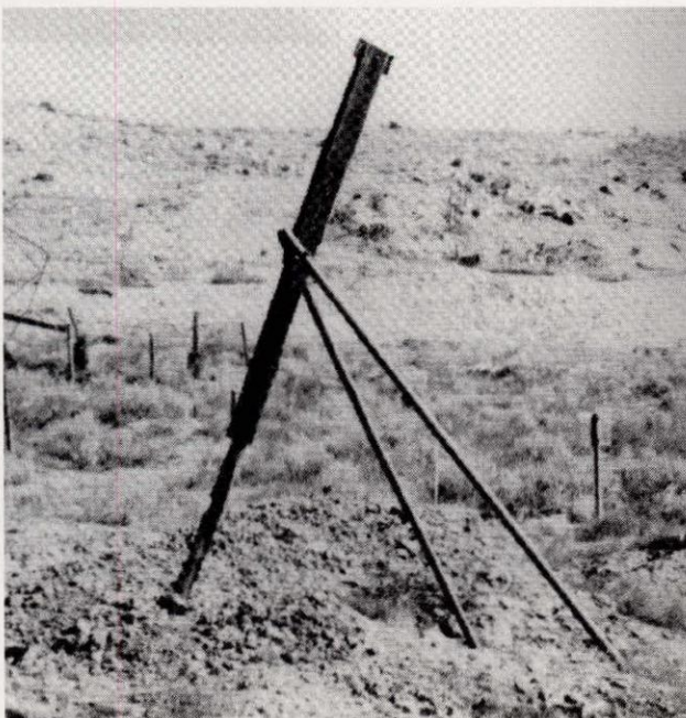
An original 'Whip Pole' built from sawn timber and steel pipes used over a mine shaft during the early part of the century near Kalgoorlie.
