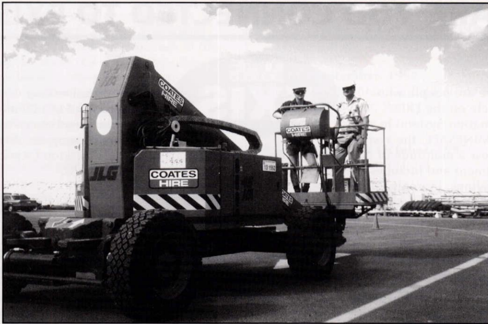
Rodney Goldsworthy (Right) training an employee to use an elevated work platform.
