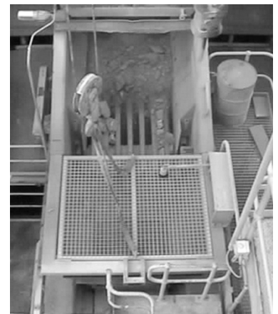
Protective grate being lowered into position over the jaw crusher
