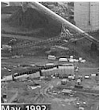
Mine surface infrastructure
