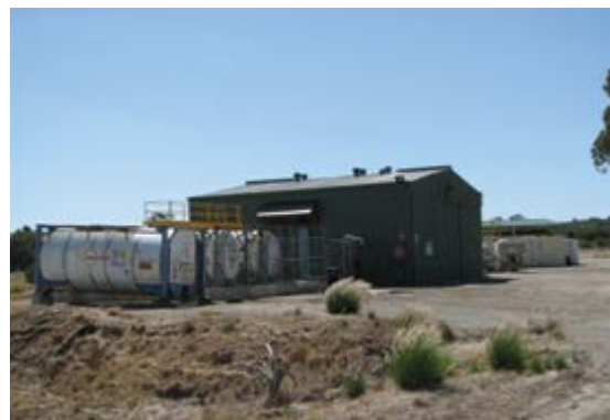
Ammonium nitrate emulsion manufacturing site
