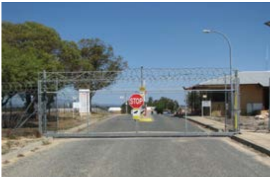
Main gate and gate house
