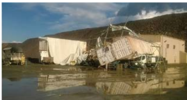
Building and temporary structure damage following severe storm events. Left. Collapse of heavy mobile plant workshop roof. Right. Overturned container shelter.
