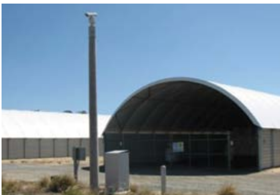
Ammonium nitrate storage and security camera
