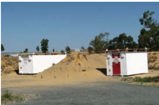
10 tonne relocatable magazines
