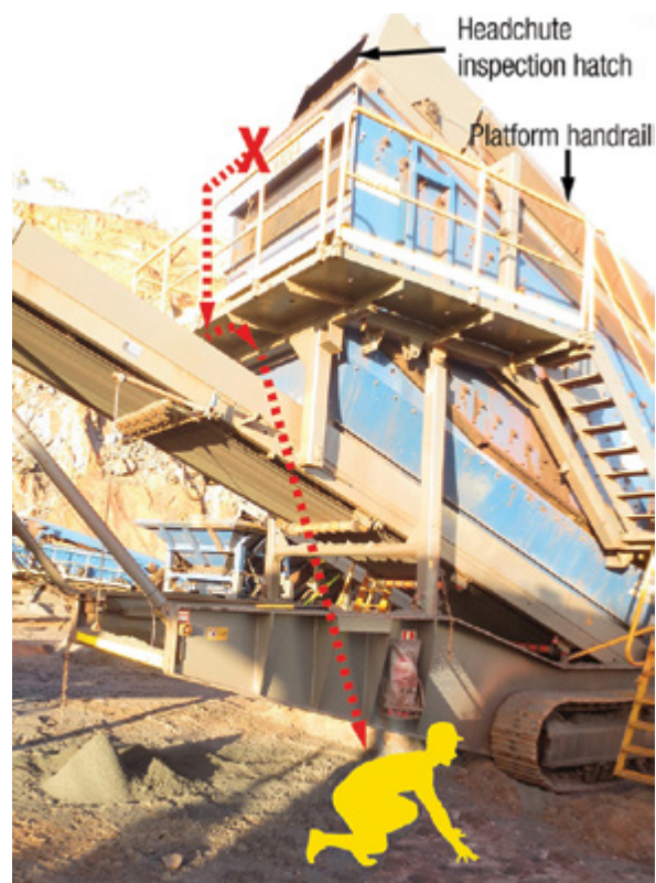
Photograph showing the location of the headchute inspection hatch on the mobile screening plant and the supervisor's fall path
