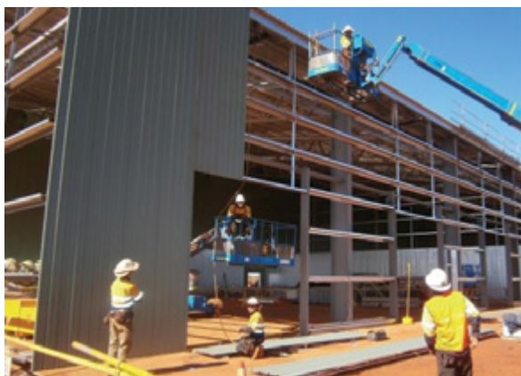
MEWPs being used in and near a structure with restricted access
