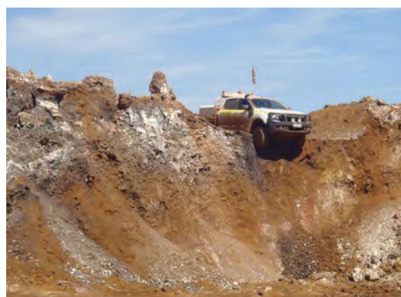
Light vehicle with front wheels hanging over open edge of excavated area
