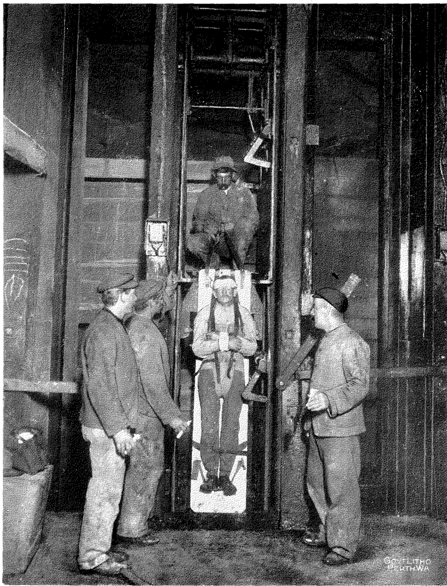
Patent Stretcher in use. Man being brought to surface in vertical position.
