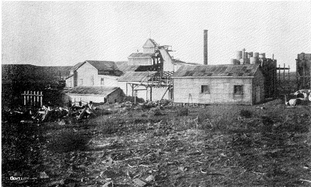
Phillips River Concentrating Plant.
