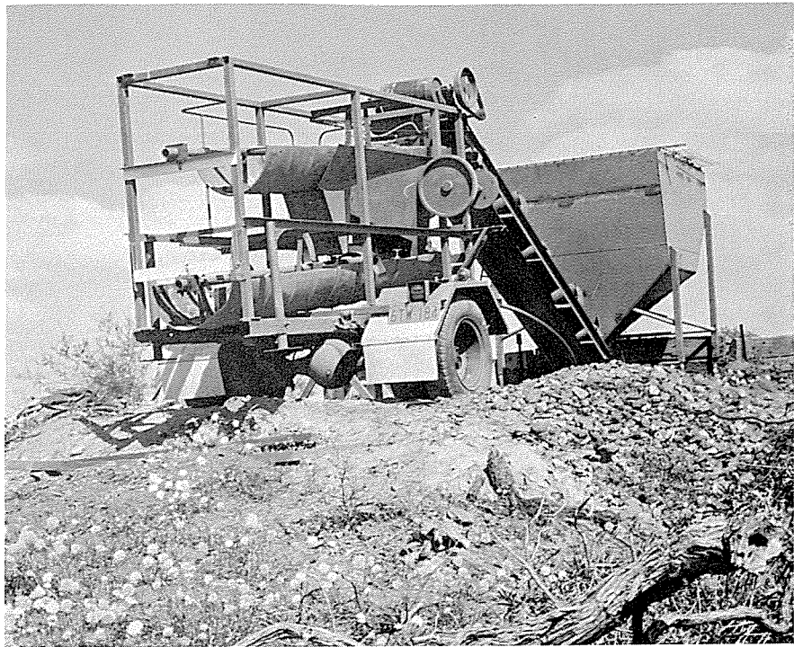
Small gravity type gold recovery plant set up on an alluvial prospect
