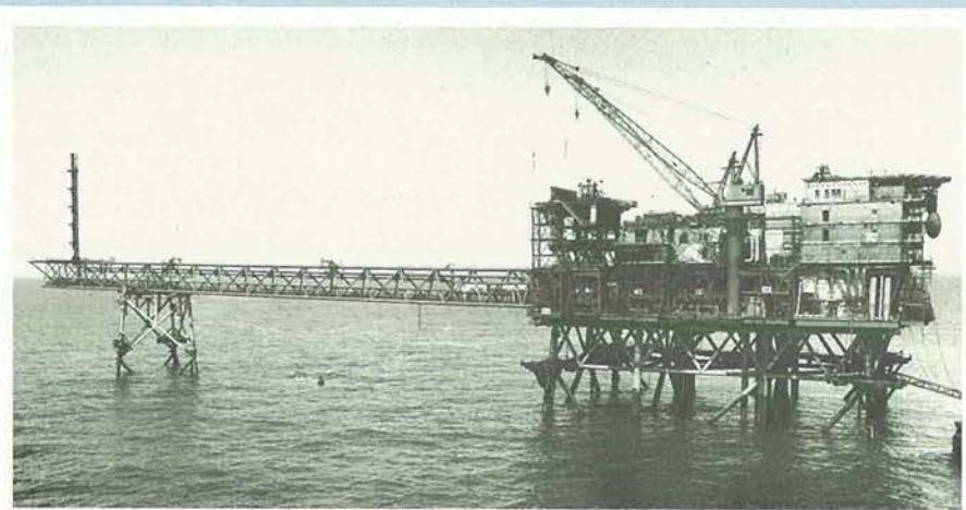
Woodside—NW Shelf Project. North Rankin 'A' platform. December 1982.
