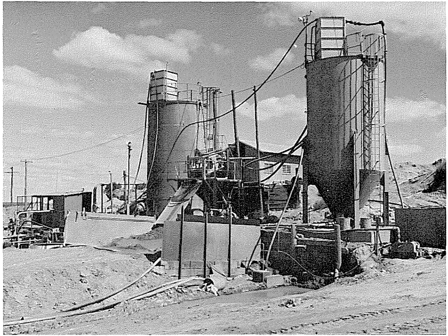
Carbon in Pulp installation, State Battery, Kalgoorlie
