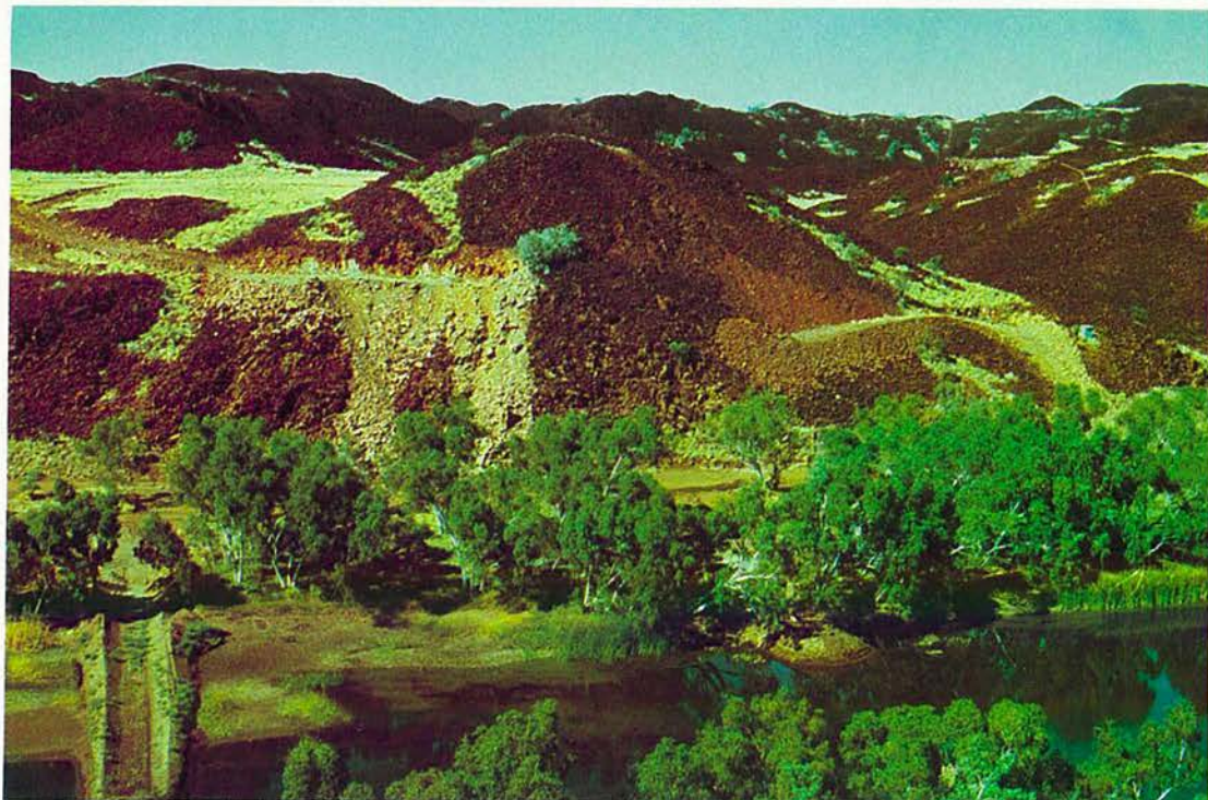
South bank at dam wall
