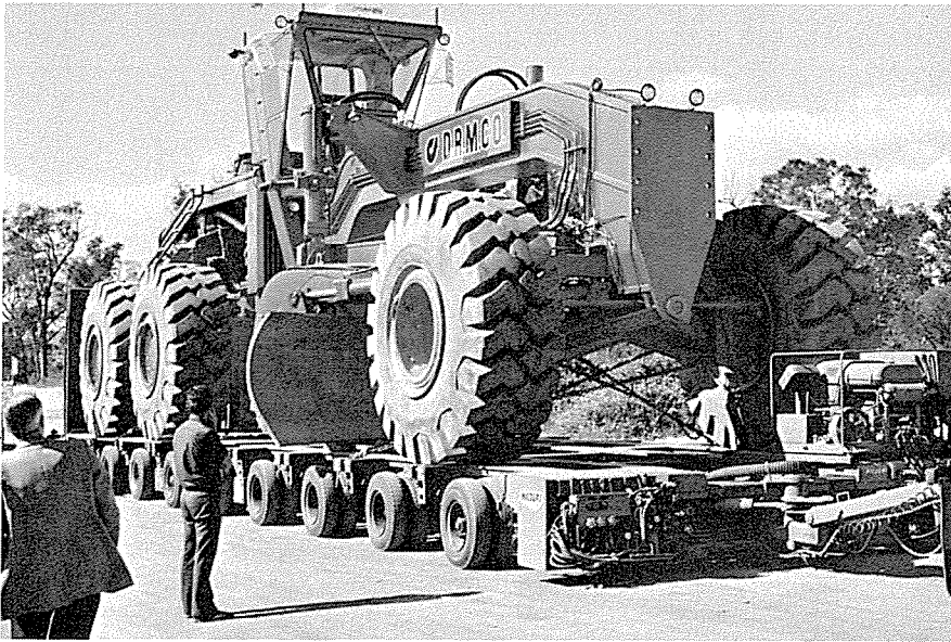
Loading a large grader for transportation to Newman
