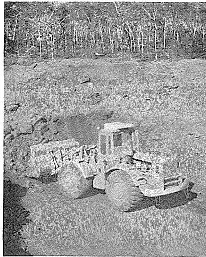
Excavating a bulk sample of bauxite on the Mitchell Plateau
