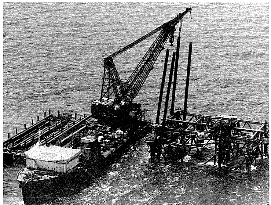
Platform piling from installation barge 'THOR' (WA Newspapers Ltd)
