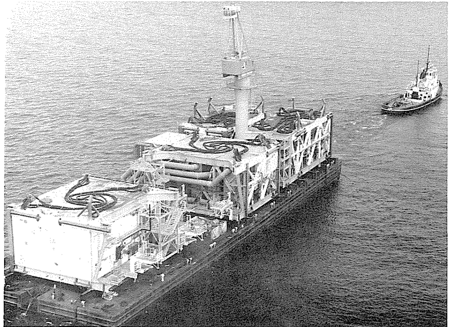
Modules under tow from Jervoise Bay to Karratha (WA Newspapers Ltd)
