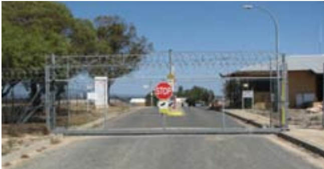
Main gate and gate house
