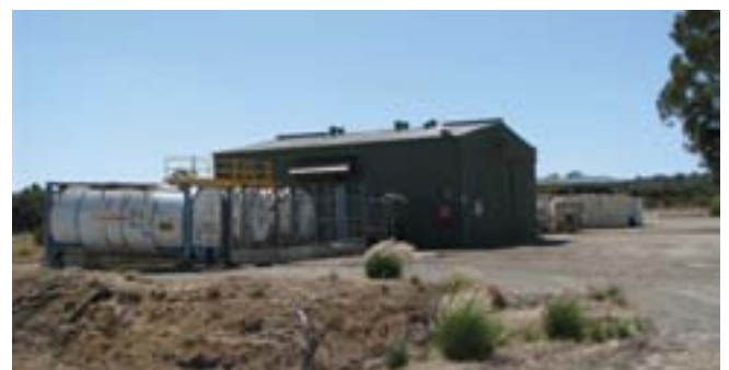
Ammonium nitrate emulsion manufacturing site
