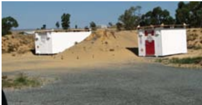
10 tonne relocatable magazines
