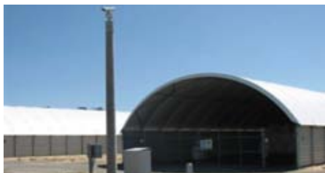
Ammonium nitrate storage and security camera
