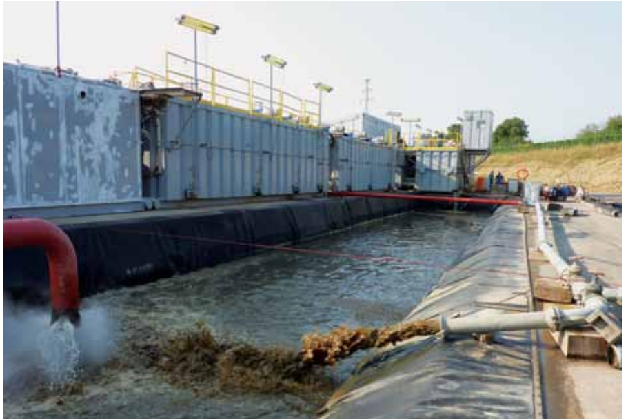
Geothermal well testing at Dr Jörg Baumgärtner's Insheim geothermal power project in Germany (Photo courtesy of Green Rock Energy)
