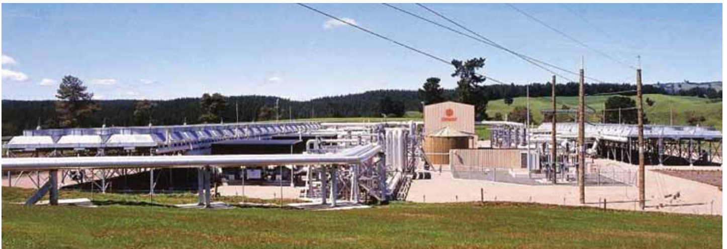
The Ormat power plant at Mokai, New Zealand — the type of geothermal power plant Green Rock Energy hope to install in the northern Perth Basin (Photo courtesy of Green Rock Energy)
