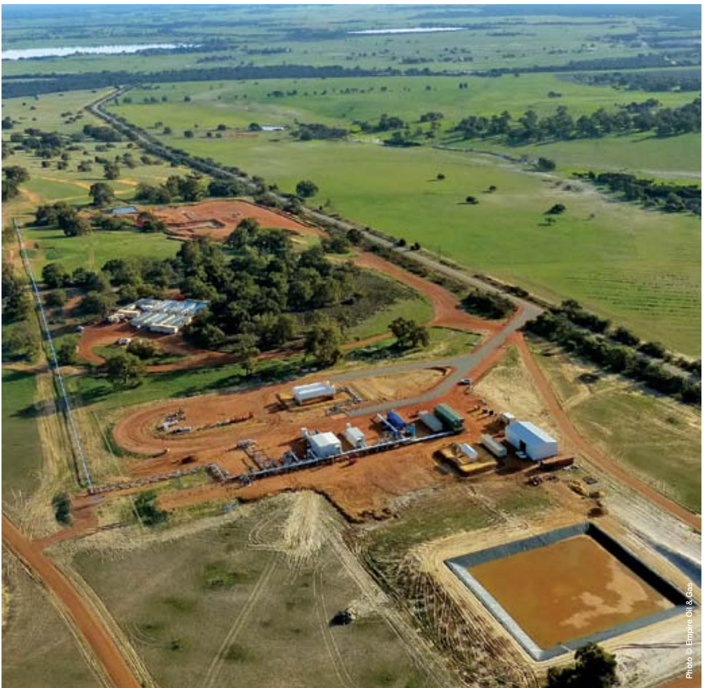
The Red Gully gas and condensate facility in the Northern Perth Basin
