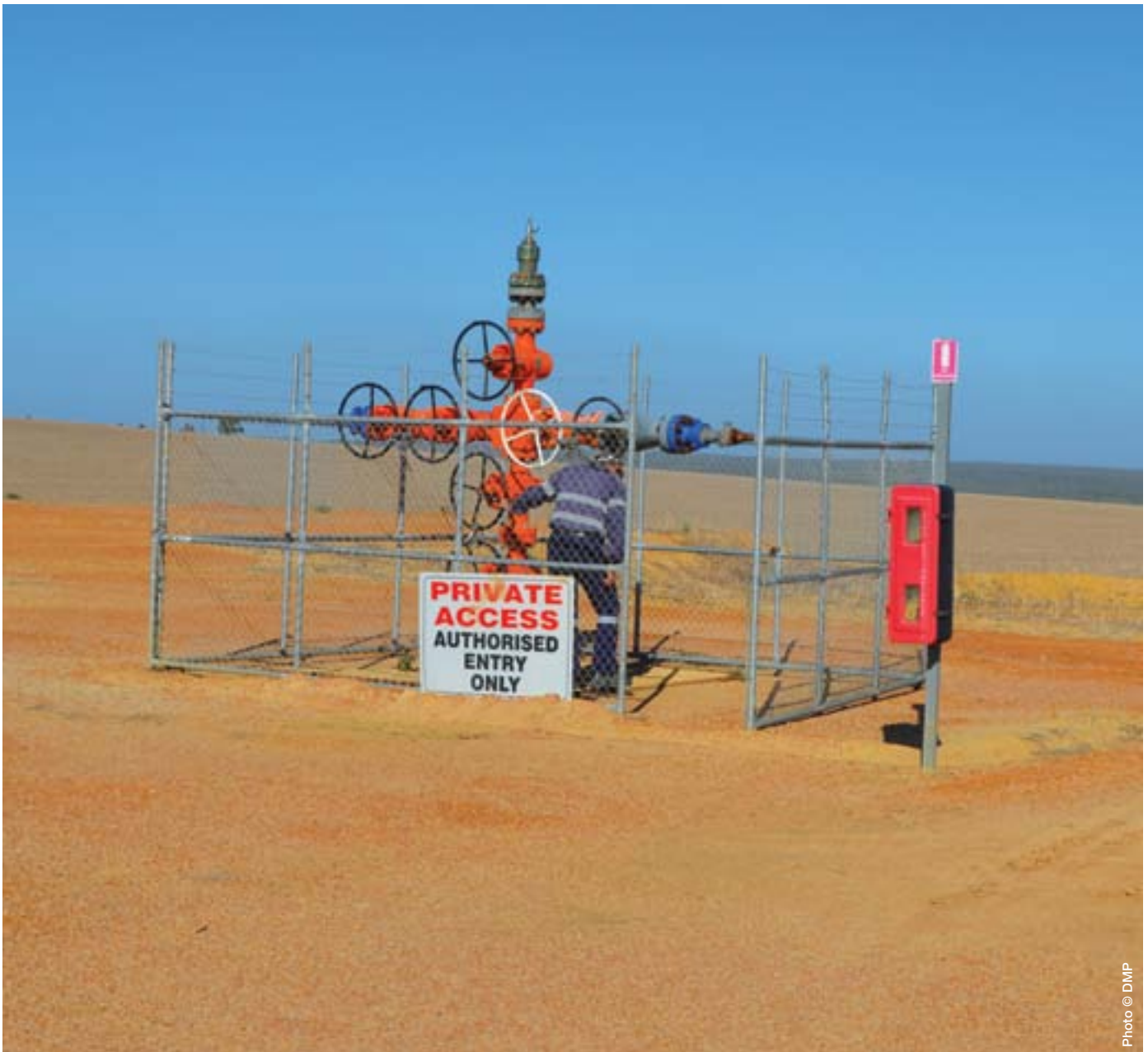
Inspection of a non-decommissioned well on the Senecio field
