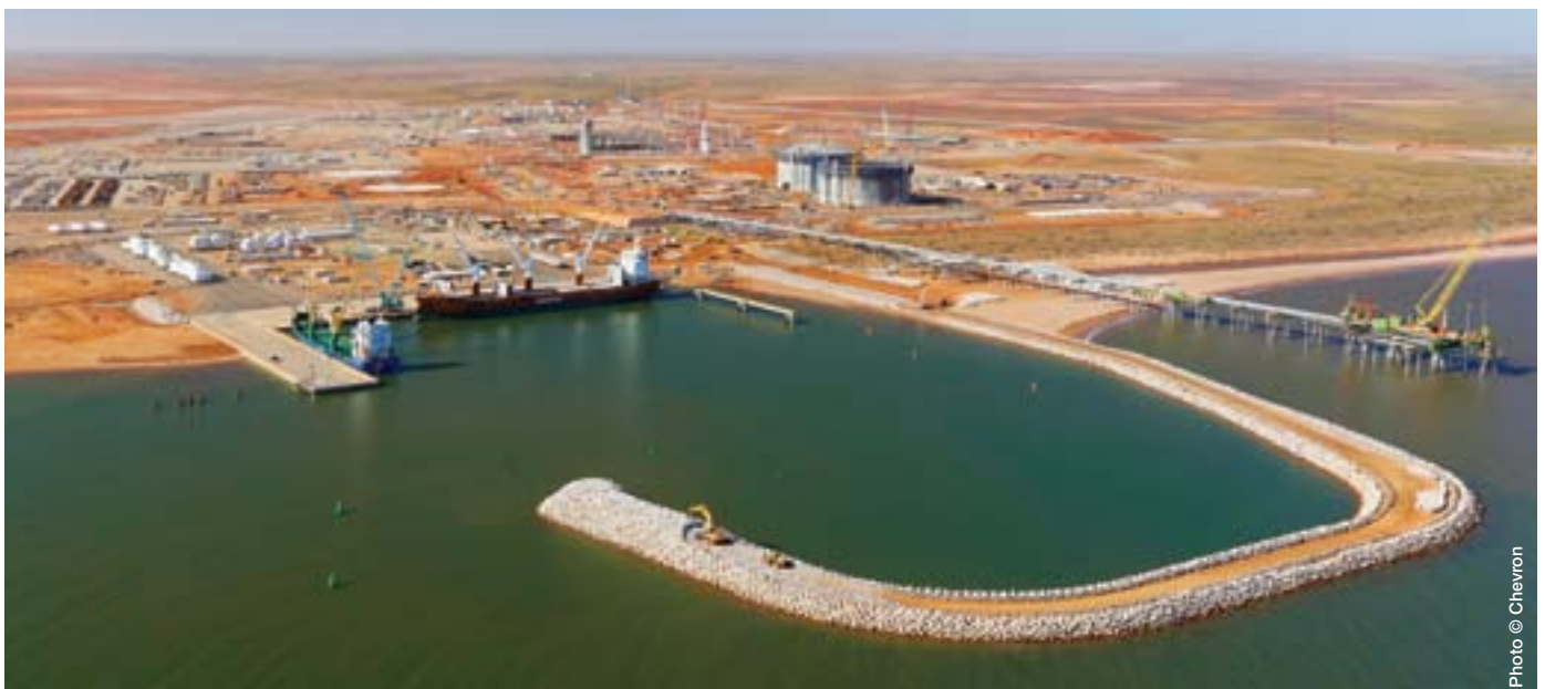
Wheatstone Materials Offloading Facility's breakwater construction takes shape
