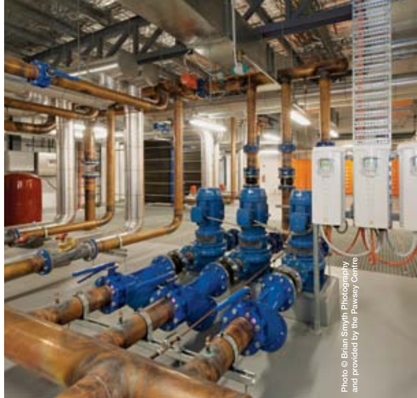
View of the groundwater cooling pumps and distribution system inside the Pawsey Centre
