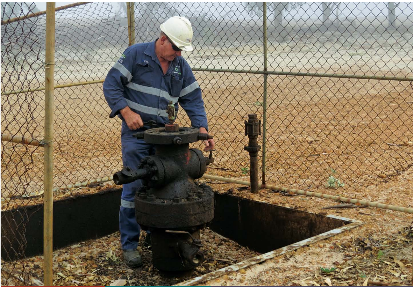
Monitoring Mt Horner 9 following well decommissioning before wellhead removal
