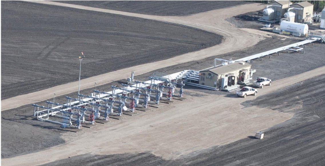
Figure 8. The area needed for a multi-well pad. This well pad in north eastern British Columbia has a total of 18 to 20 operational shale gas wells [Source: Council of Canadian Academies, courtesy Nexen Energy ULC]
