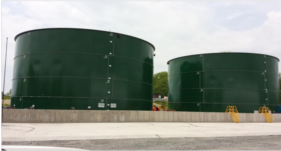
Figure 25. Cabot Oil and Gas Corporation holding tanks with wastewater to be reused for hydraulic fracturing, Susquehanna County, Pennsylvania, USA [Source: Committee site visit, 27 May 2014]
