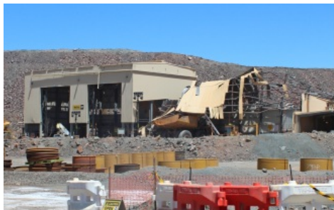
Building and temporary structure damage following severe storm events. Left. Collapse of heavy mobile plant workshop roof. Right. Overturned container shelter.
