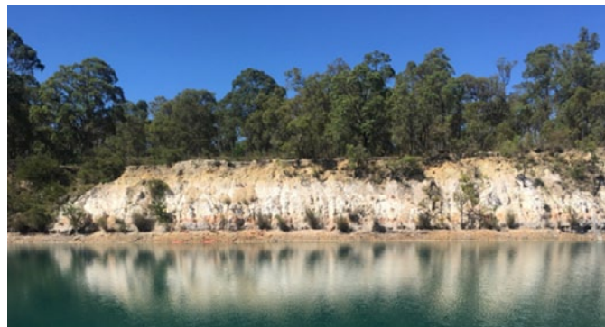
Figure 1. Southern pit wall prior to earthworks
