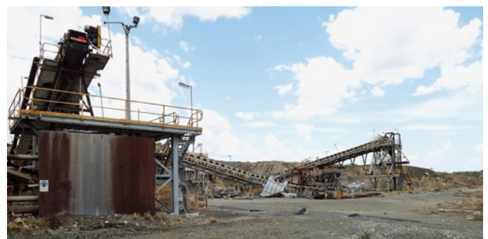
Ellendale 4, showing part of the remaining abandoned plant area
