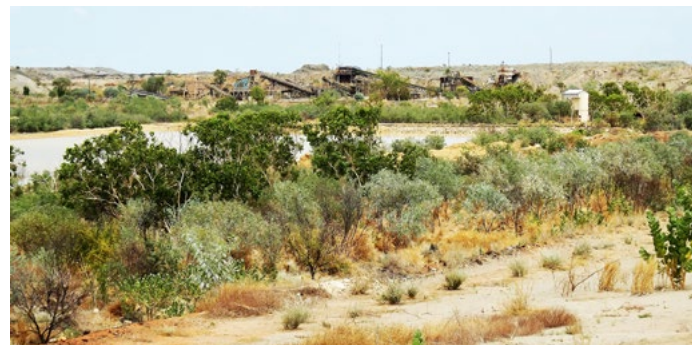
Ellendale 9 plant area looking across process water pond
