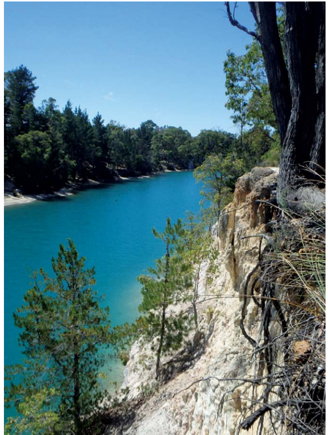
Steep pit wall at the abandoned Black Diamond Pit Lake. Source DMP 2016
