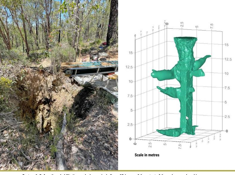
Feature 8: Before the rehabilitation works begun, including a 3D image of the extent of the underground workings.
