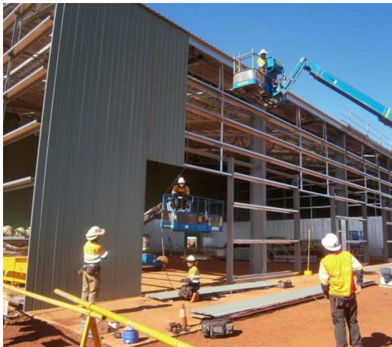
MEWPs being used in and near a structure with restricted access
