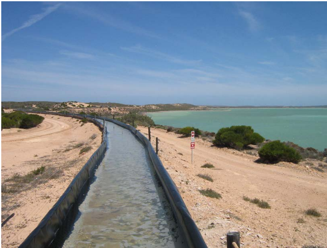
Plate 4: Water flume, electric fence and overhang to deter fauna, (Shark Bay Salt JV).
