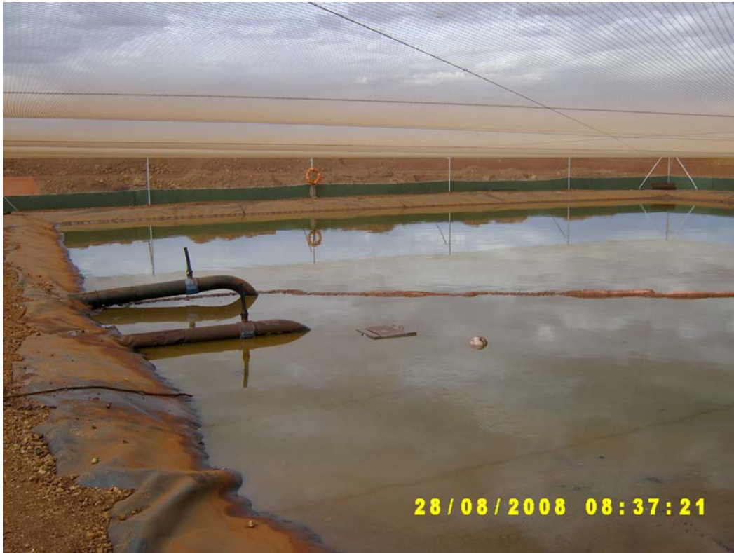
Plate 3: HDPE pond netted and fenced to exclude wildlife (Fortescue Metals Group, Cloudbreak).
