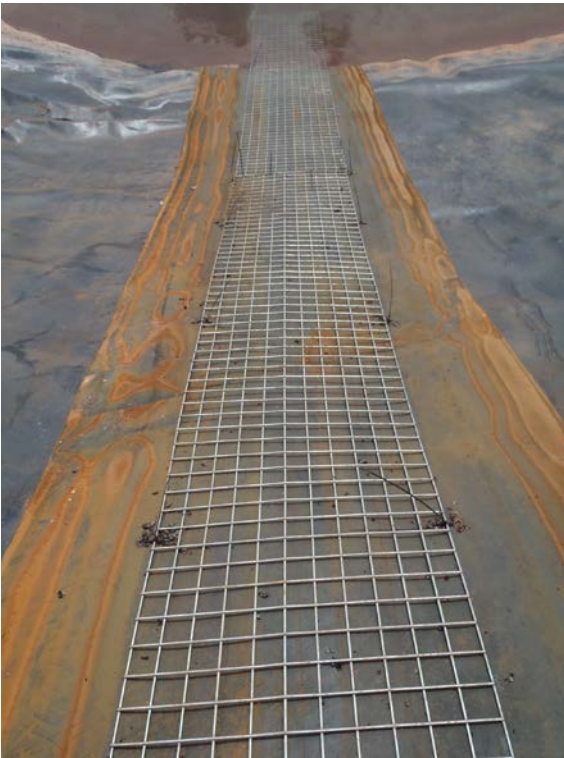
Plate 5: Example of successful fauna egress using conveyor matting and a mesh stripe which is firmly secured to the matting with cable ties (BC Iron Nullagine Pty Ltd).
