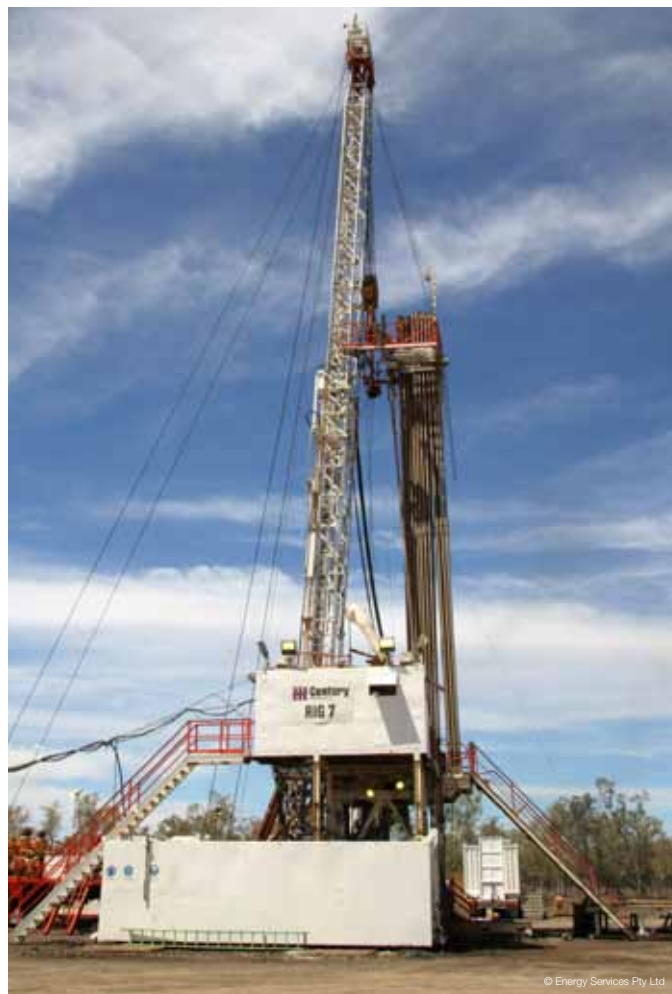
The Century Rig 7 which will be used to drill the Harvey 1 Well.
